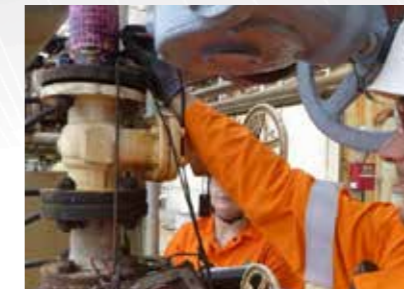
Non-Destructive Testing (NDT)
