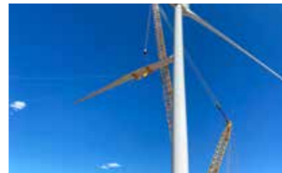
BLADE REPAIR & REPLACEMENT
